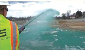
FINN invented the HydroSeeder® in 1953 creating a new industry of turf and erosion control contractors. Hydroseeding is far more efficient than broadcast seeding or installing sod. It speeds the seeding process, saving time, labor hours and money. And the results are lush, thick grass beds that establish quickly.
