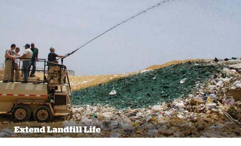
Each cubic yard of dirt that is used for daily cover results in a permanent loss of revenue on space that cannot be sold. FINN's Alternative Daily Cover takes up 24 times less space than dirt, extending the life of the landfill.
