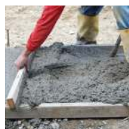
Driveway / Sidewalk Contractors
