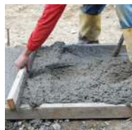
Driveway / Sidewalk Contractors
