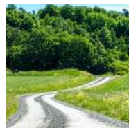
Gravel Road Maintenance
