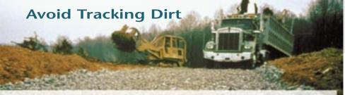
Design construction site exits to limit the tracking of dirt and other pollution out of the site. An ideal site exit includes use of a tracking pad.
