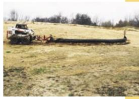
Silt-fence installed using the slicing method results in minimal soil disturbance and produces less washouts compared to trenching.
